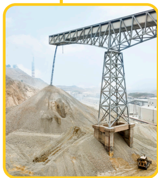
Implementation of concrete foundation and metallic structure for the conveyor belt number 2
